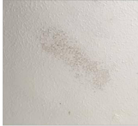
Photo - 31 Dirt/mould
