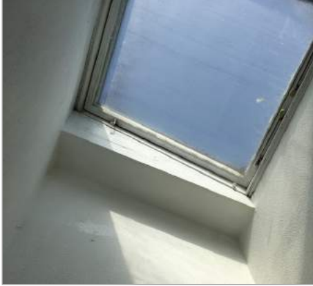
Photo - 9 Maintain/replace roof light
