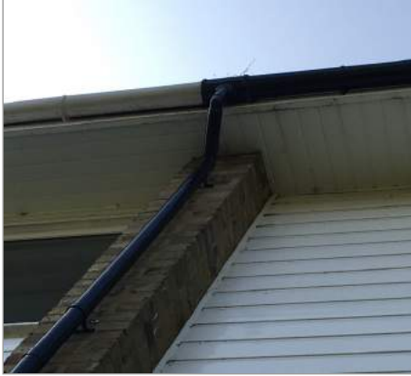
Photo - 2 Remove vegetation from guttering
