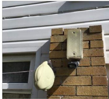
Photo - 8 Repoint rear pier
