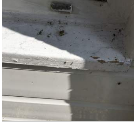
Photo - 10 Maintain timber frame
